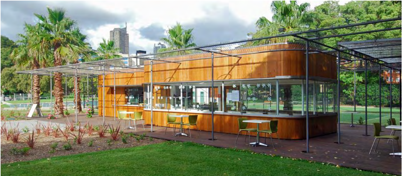
KIOSK – BLACKBUTT CLADDING (CURVED WALLS)
