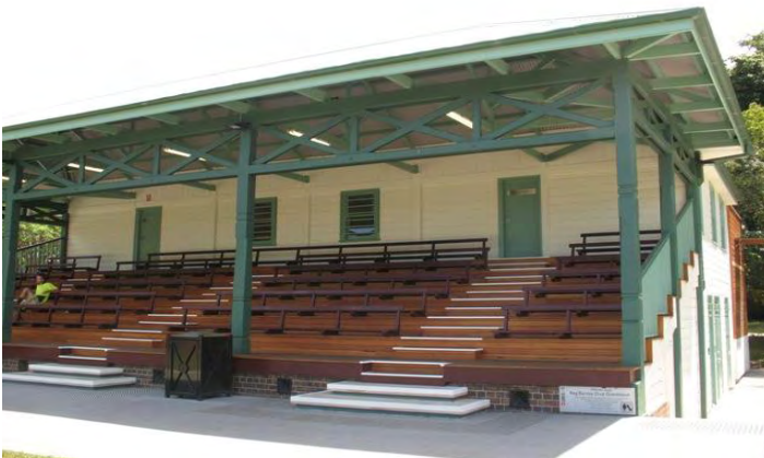
GRANDSTAND HERITAGE CLADDING & STRUCTURAL TIMBERS
