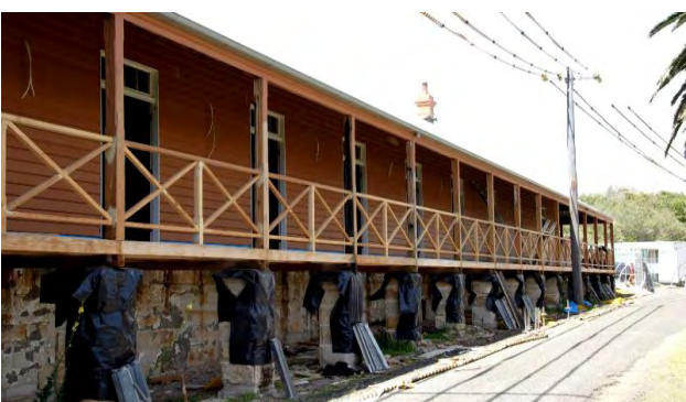
BUILDING P22 – DURING RE-CONSTRUCTION (NOV 2006)
