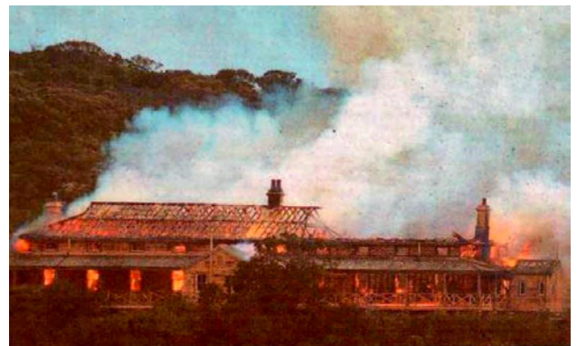
BUILDING H1 GUTTED BY FIRE (FEB 2002)
