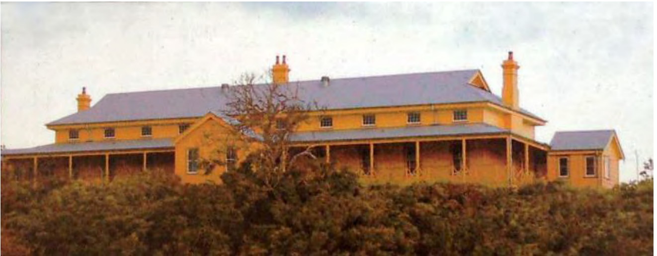
NEW BUILDING H1 – RESTORATION COMPLETED (2007)
