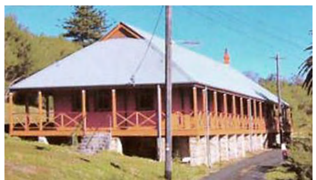
RESTORATION COMPLETED - BUILDING P22 (2007)
