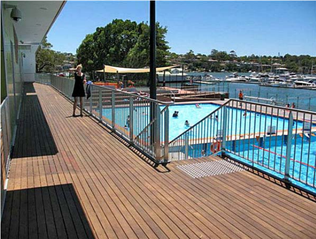
86 X 19 TURPENTINE – CABARITA SWIMMING COMPLEX
