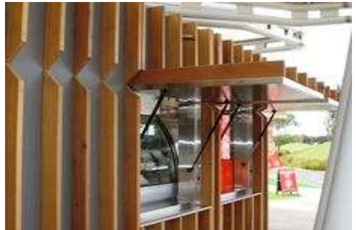
TIMBER FINIS CUT TO SIZE & OILED IN FACTORY
