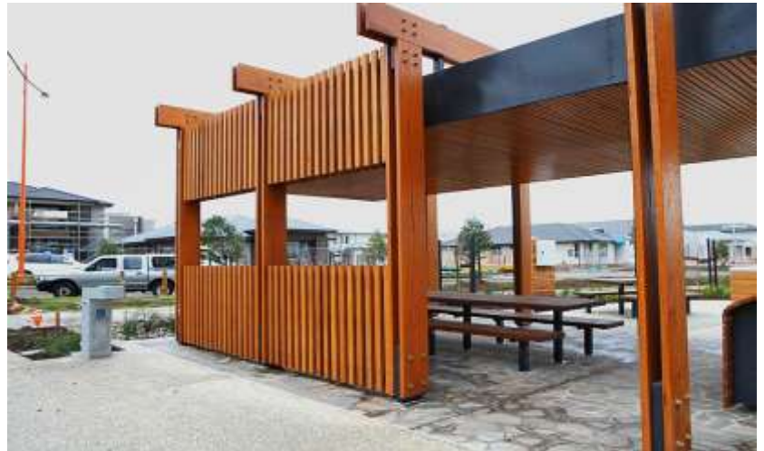
BLACKBUTT POSTS, SCREEN WALL & BEAMS
