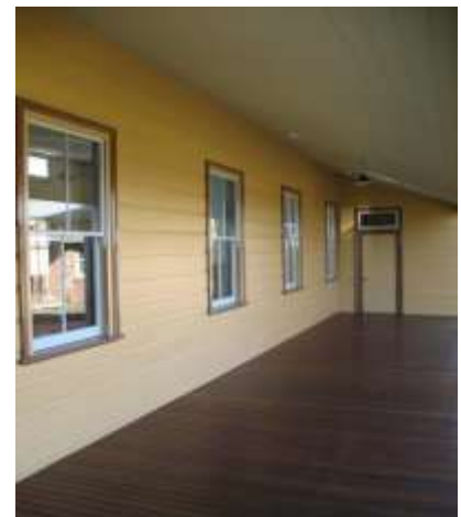
BLACKBUTT CEILING PANELLING
