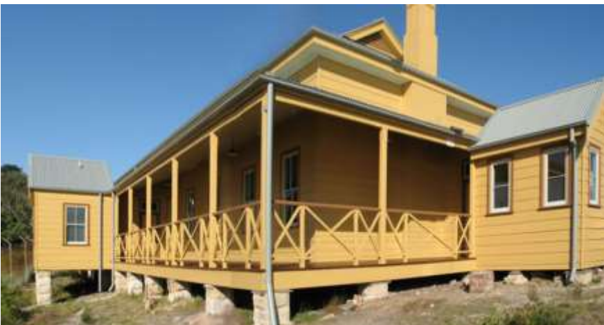
BLACKBUTT BALUSTRADE AND HANDRAIL
